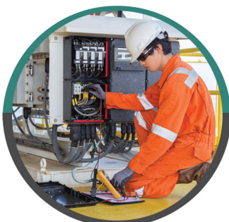
Panel Installation & Commissioning
